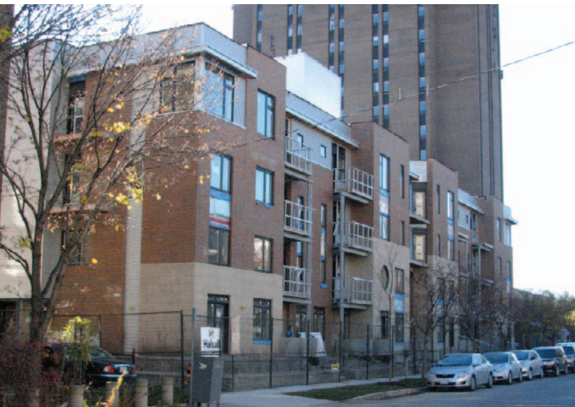
160 Argyle, Phase 1, 4-storey apartment looking west at the north elevation
